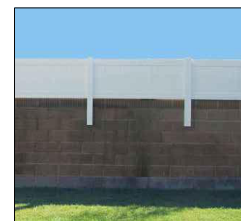
CONNECTION DETAIL 2' HEIGHT VINYL FENCE EXISTING 6' HT MASONRY WALL
